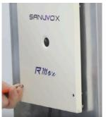
11. Secure the R Max to the frame with the 4 remaining screws located in the 4 corners of the R Max cover.
