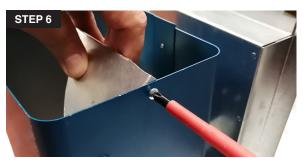
6. Once the UV lamp is installed, place the turbulator inside the reflecting chamber securing it with 3 screws provided in the installation kit. It is important to note that the air should first flow through the turbulator before moving in front of the UV lamp.
