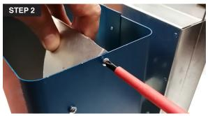
2. Remove the turbulator to access the lamp.
