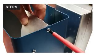
Once the new UV lamp is installed, replace the turbulator inside the reflecting chamber, and replace R Max into duct.
