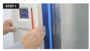
1. Take the R Max out from the ductwork by removing the 4 screws located on the cover (4 corners) that hold it to the frame.
