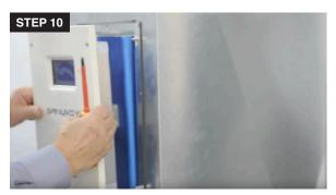
10. Finalize the R Max installation in the duct by placing the unit into the frame, guided with the alignment pins.
