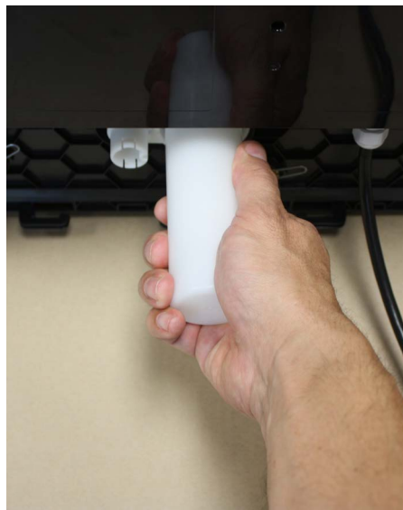
Figure 17: Condensate trap installation
